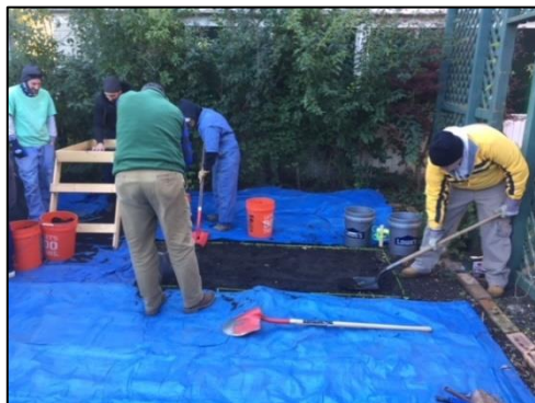
Figure 5, Initial opening of unit
