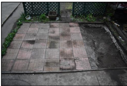
Figure 30, Unit6 5 & 6 before excavation
