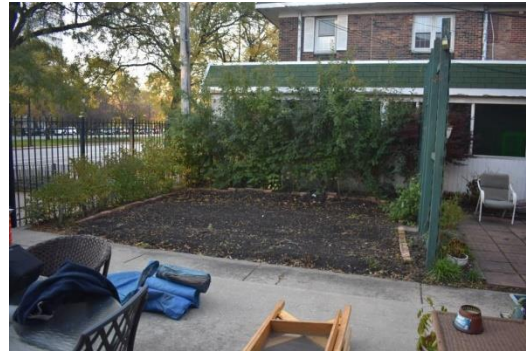
Figure 4, Site after excavation and backfill
